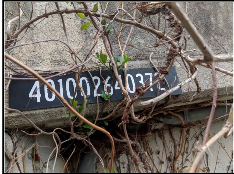
2 The bridge is identified as structure # 401002640372.
